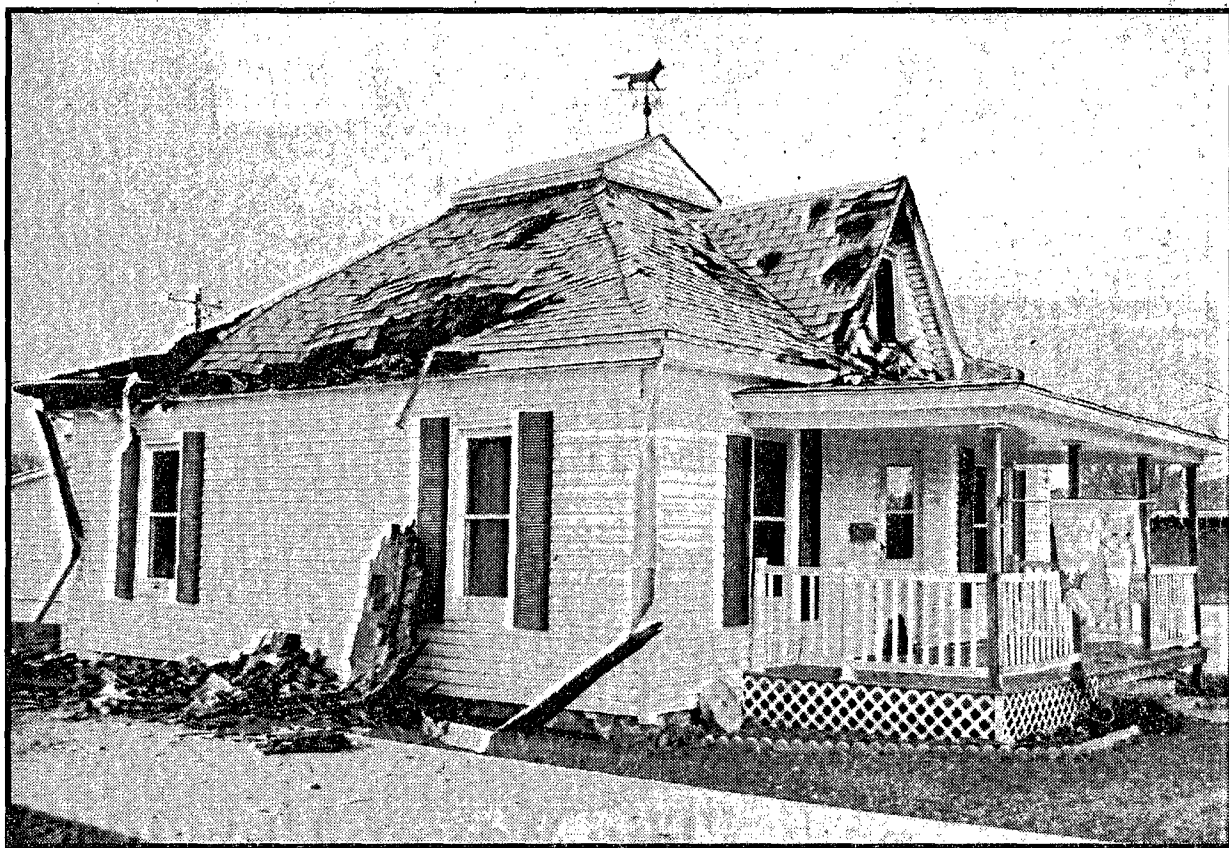
A fire destroyed this home last Thursday night. Both the Wayne Volunteer Fire Department and the Carroll Volunteer Fire Department responded to the call at 428 East 4th Street in Wayne.
